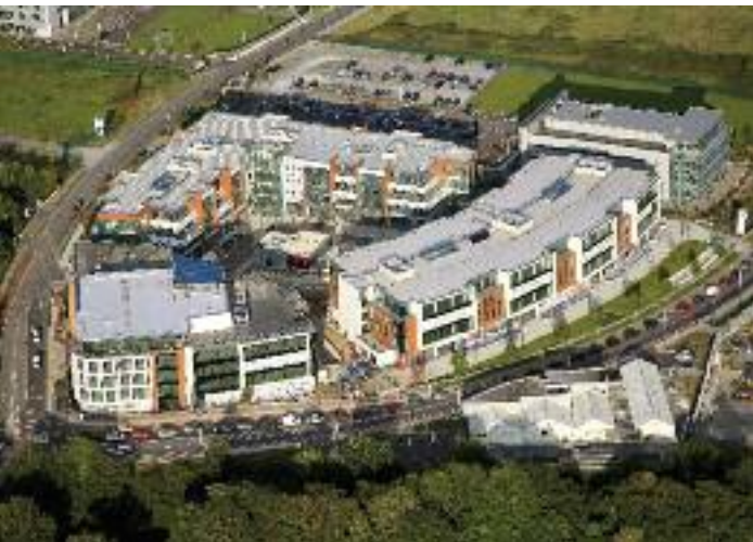
City Gate Mahon , Cork_Ireland. product installed: CBH Fully Steel Encapsulated Panels 31 mm. surface: 35.000 sqm.
