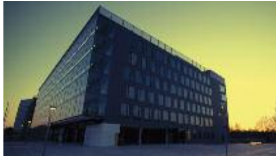
Gerechtsgebouw , Ghent_Belgium product installed: fully steel encapsulated panel. surface: 28.000 sqm. design: Stéphane Beel Architects.
