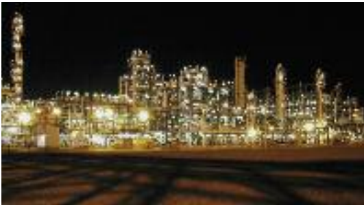
National Chemicals Co Chemawajaat Offices , Abu Dhabi_UAE product installed: fully steel encapsulated panel. surface: 8.500 sqm.
