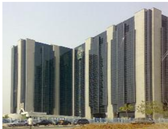
Central Bank , Abuja_Nigeria. product installed: calcium sulphate panel high density 34 mm > top covering linoleum. surface: 15.000 sqm.
