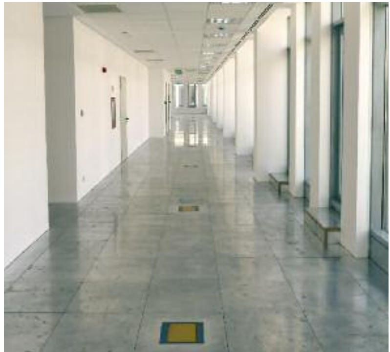
double alufoil panels › woodcore calcium sulphate 34 mm › Swan Office Park_Bucharest (35.000 smq)
