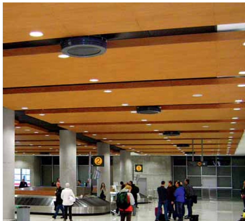
Sherwood Melamine › cherry › perf. A11 / wood concealed 200 system CWI 100% removable with special suspension system CBI Europe Larnaka Airport _ Cyprus
